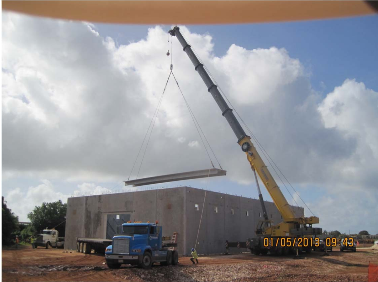
PRE-CAST CONCRETE DOUBLE TEE (WITH CONCRETE TOPPING)
