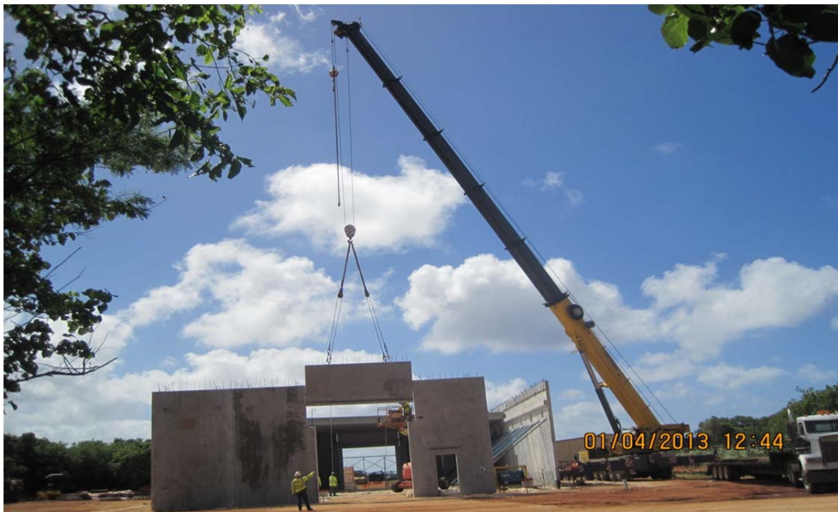
PRE-CAST CONCRETE DOUBLE TEE (WITH CONCRETE TOPPING)
